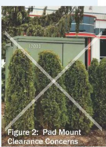
Figure 1: Clearances to Pad Mounted Equipment
