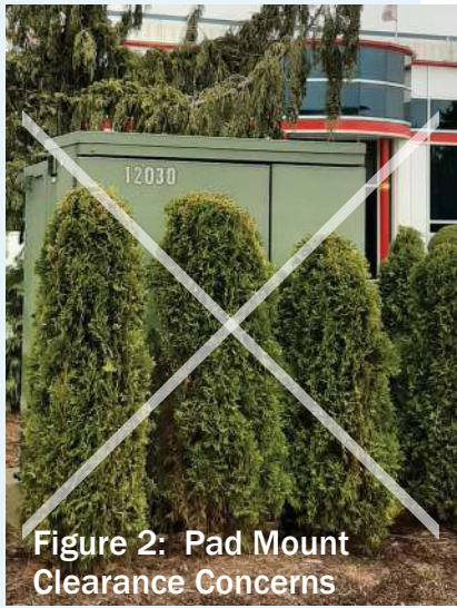
Figure 1: Clearances to Pad Mounted Equipment
